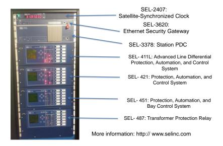
Fig. 4: Phasor Measurement Unit Rack - Four PMUs.
